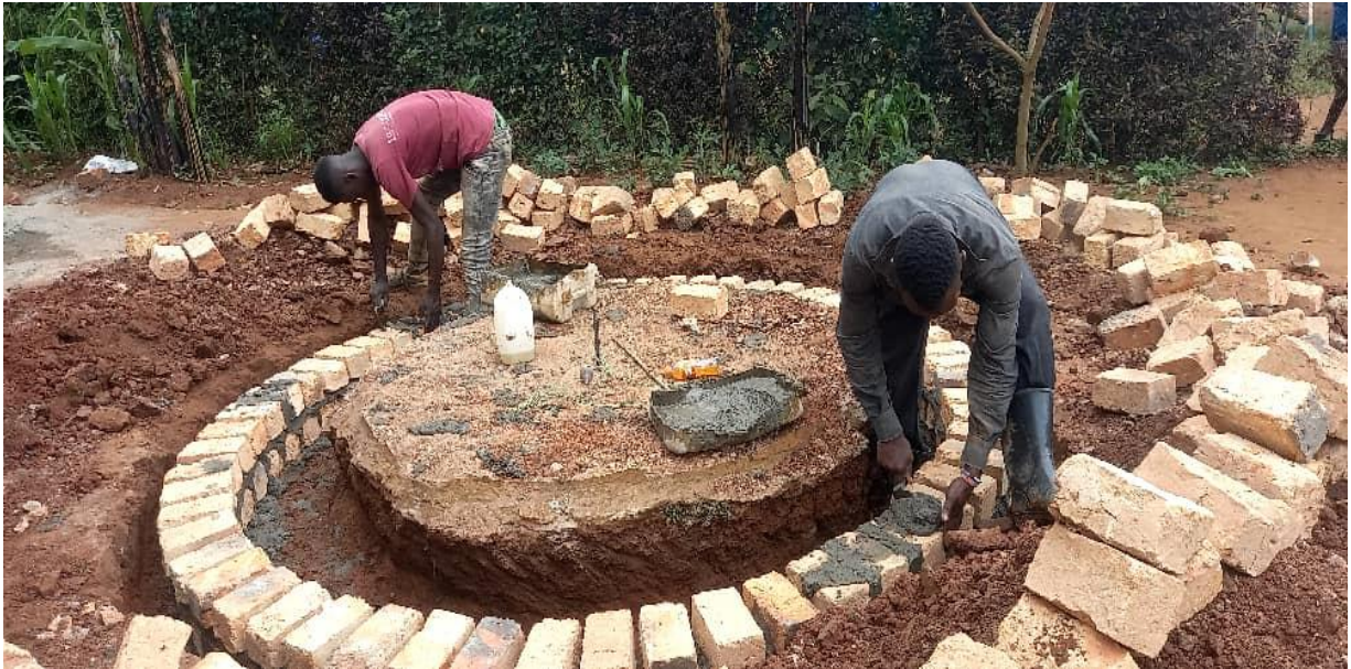
Construction of the tank basement being done at Kitezi Primary school-Uganda
