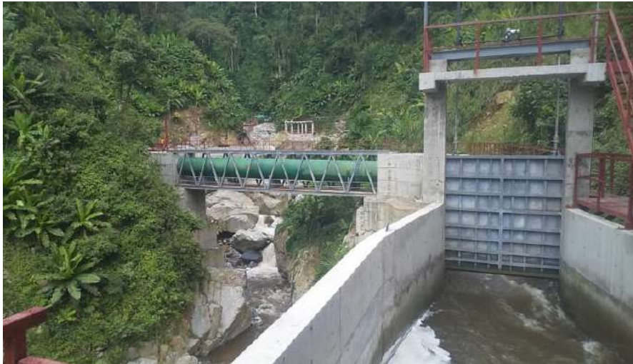
Figure 2: Nyamugasani 1 Hydropower intake
