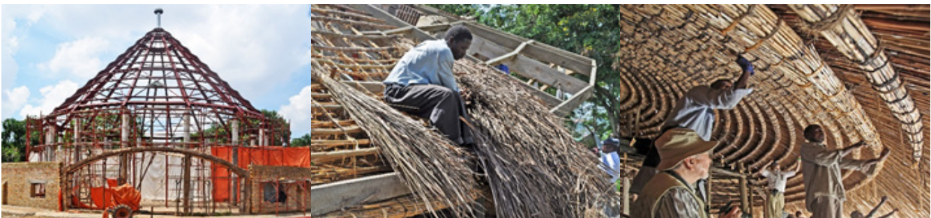
Raised part of the structure
