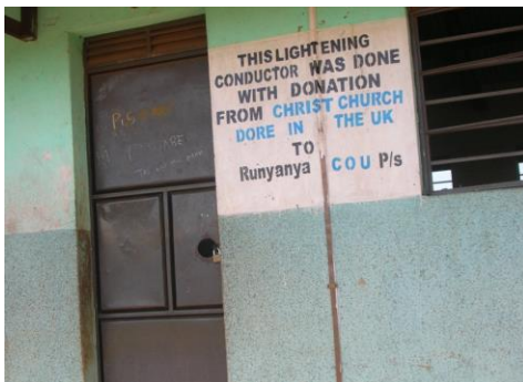
Plate 5.9. The commissioning of the lightning conductors at the school.
