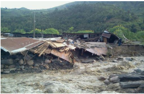
Plate: 2.7. Houses destroyed by floods in Kilembe
