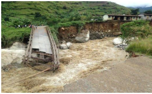
Plate 2.4: Washed away bridge connecting to Kyanzuki and Kilembe SS (36N0166816 UTM0022310). Photo credit: Kitutu Goretti
