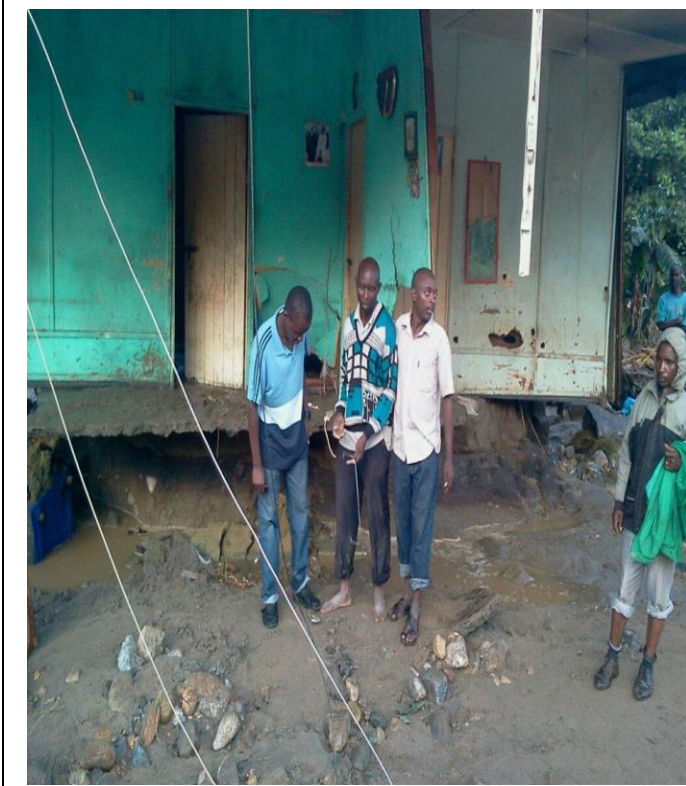
Houses damaged by floods. The houses now stand on pillars.
