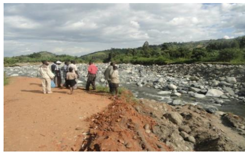
Plate 2.6: River Mubuku destroyed the road and went back to the 1961 course. Photo credit; Kitutu Goretti
