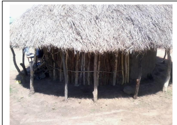
Plate 2.11. A house being renovated with poles after the wall was damaged by floods, 2013: Photocredit: Dr. Kitutu Goretti
