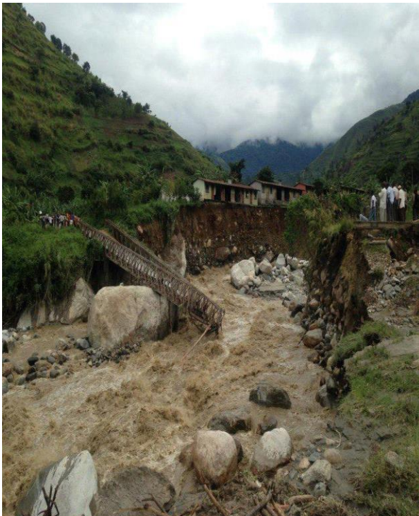
A broken bridge in Kilembe. Transport was greatly affected.
