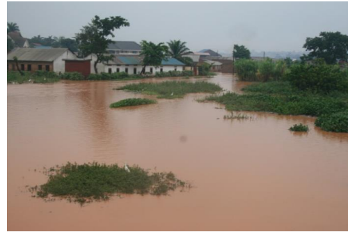
Plate 2.24: Houses sub-merged in floods in Nsooba -Kalerwe areas (3/5/2013)
