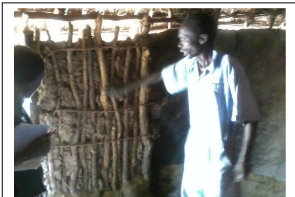
Plate 2.10. Akinde LC1 chairman explaining the effects of floods and the new method of constructing houses using poles. Photo credit : Dr. Kitutu Goretti 2013.
