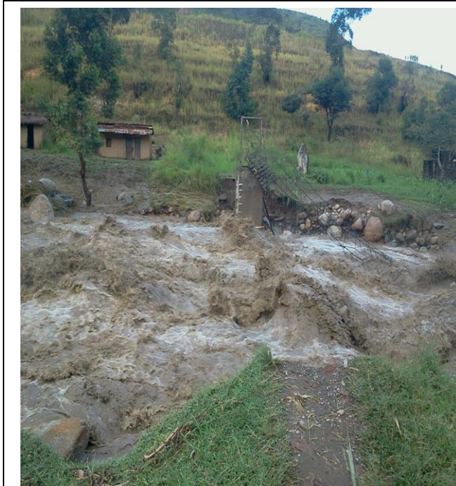
Broken bridge caused by too much water pressure and debris
